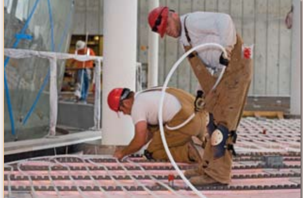
In installing a radiant floor system, spacers are used to assure the correct heat density in each area. This can be varied for varying climate conditions and differing uses of spaces.
