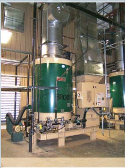
Whether it's new construction or a retrofit, owners appreciate the small footprint of a coil tube boiler, as with this Clayton compact vertical unit in a grain processing plant. Photo courtesy Clayton International.
