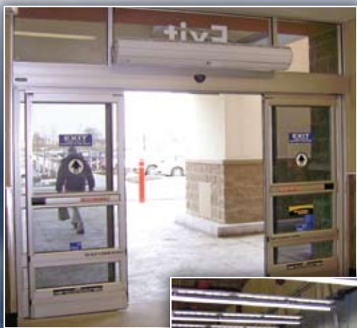
◆ Long rows of loading dock doors can be individually protected with air curtains that switch on when the door is opened. Photo courtesy Enershield.
