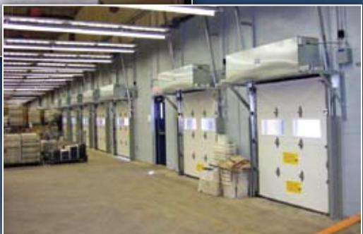
◆ Long rows of loading dock doors can be individually protected with air curtains that switch on when the door is opened. Photo courtesy Enershield.
