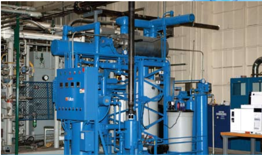
This skid-mounted boiler package from Fulton Boiler Works is the type of unit that is used for dedicated service for steam humidification in an industrial facility. Photo courtesy Fulton Boiler Works
